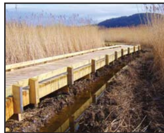
Completed boardwalk March 2009
